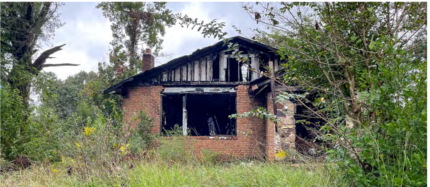
Image 2.1 Abandoned house on Lloyd Nolan Parkway
