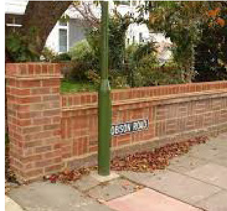
BRICK MASONRY SITE WALL
