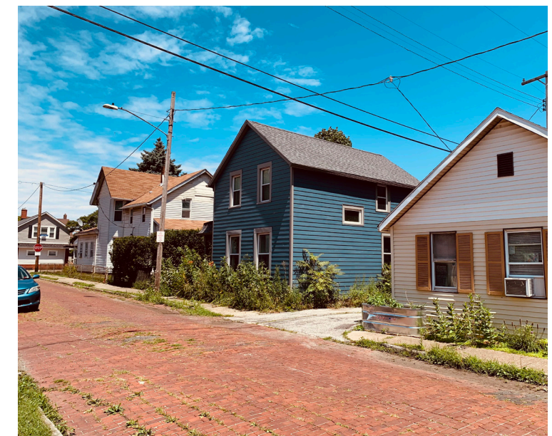
Multiple frontages. Corner lots have at least two primary street frontages. Here is a great local example of how buildings can be organized on a single or split parcel to address both street and an alley
