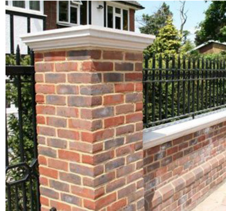
BRICK MASONRY SITE WALL W/ METAL FENCE INFILL
