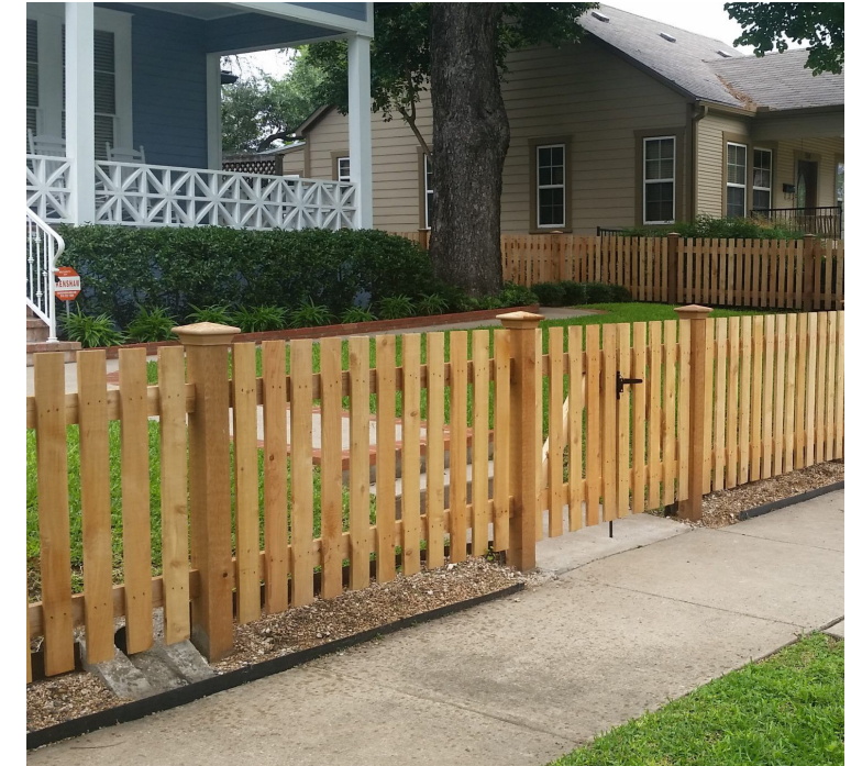
VERTICAL WOOD FENCE W/ GAPS BETWEEN PICKETS FOR OPACITY
