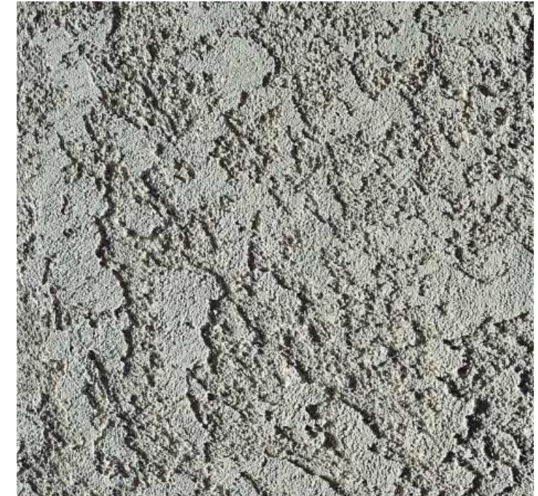
STUCCO VENEER THREE COATS OVER WIRE MESH
