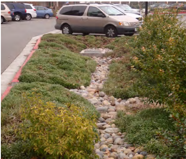
Image 5.14 Dry swale (epa.gov)
