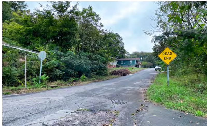
Image 5.2 52nd St. pavement condition
