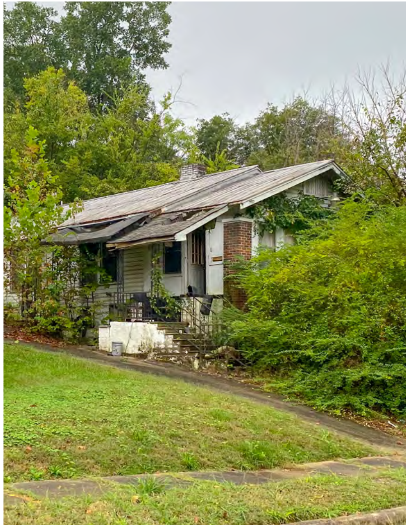
Image 6.2 Vacant House, 54th St.
