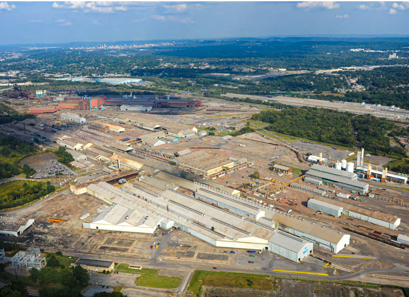
Image 7.5 U.S. Steel Fairfield Works
